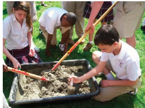
Eighth graders Morgan Boston, Naafee Rone, and Vincent Ruffini stir the cement to be used in the first reef ball constructed through our grant with the Chesapeake Bay Trust Foundation.
